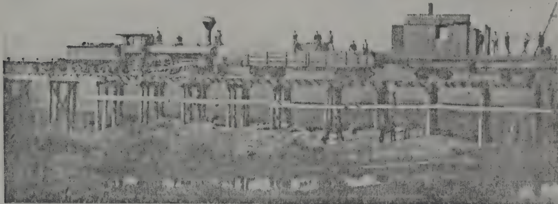
This picture supplied to us by Mrs. Bertha Long Jones bears her father's stamp on the back, "W. R. Long, Landscape Photographer." It was taken somewhere north of town while the Milwaukee Railroad was under construction, back in 1884. As everyone knows, railroads must have a fairly level track. This means cutting down the high places or building up the low. In the past, a favorite way of building up the low places was by means of an elevated wood framework known as a trestle. The construction train and crew are here shown on such a trestle. Many trestles have since been replaced by fill-ins of dirt, as has been the case of the scene of this picture.
